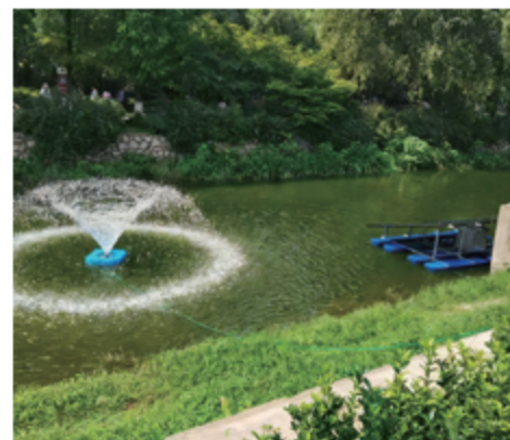
Solar Fountain Aerator Installation Site
