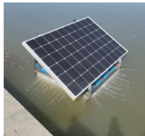
Solar Micro-nano Aerator Installation Site
