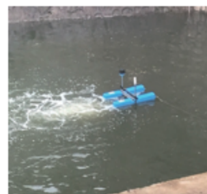
Push-flow Aerator Installation Site
